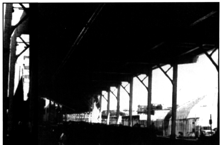
Figure 3. Whitehurst Freeway Elevated Structure
